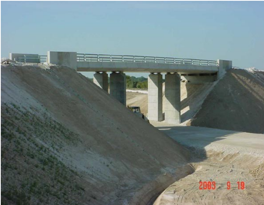
Pont-Route (Photo FNTF)
